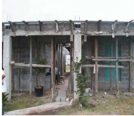
House under construction
