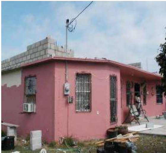
Building second floor
